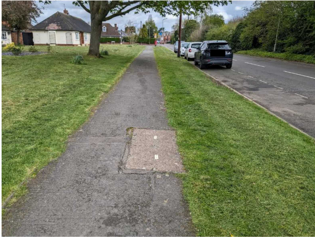
Route 1: Cross Road Footway/Verge
