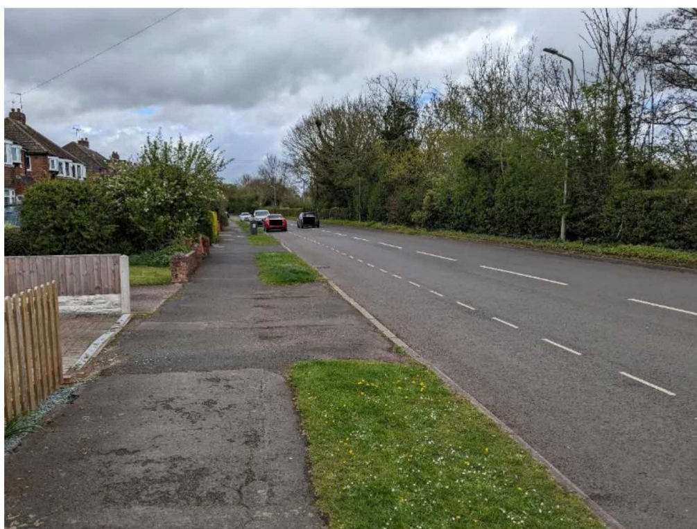
Route 1: Cross Road Footway/Verge
