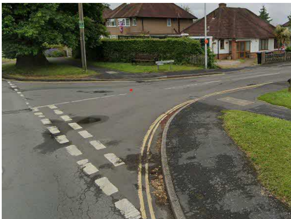
Route 3: Station Road junction with Brooklands Road
