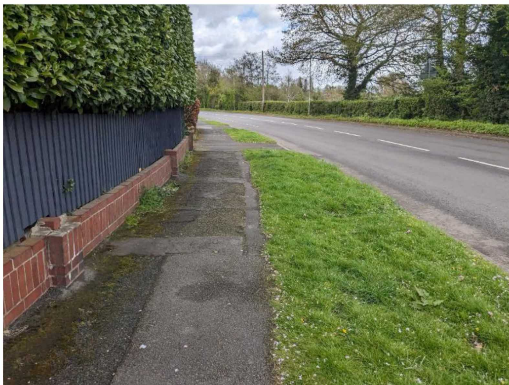
Route 1: Cross Road Footway/Verge
