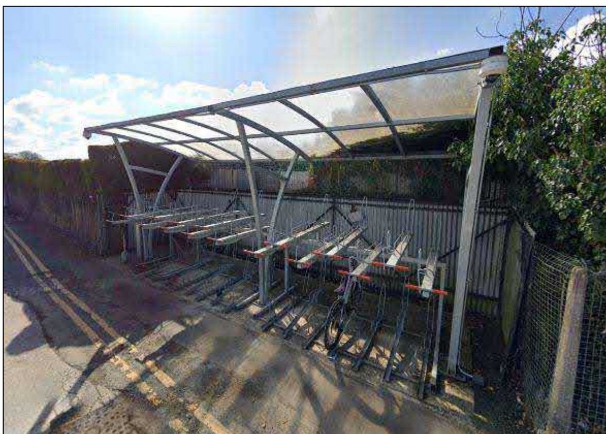
Figure 14. Cycle Parking at Albrighton Railway Station (CCTV Monitored)
