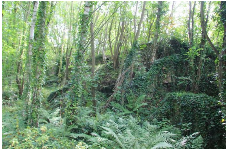
Figure 17 Part of the remains of Tong Castle as seen from the east
