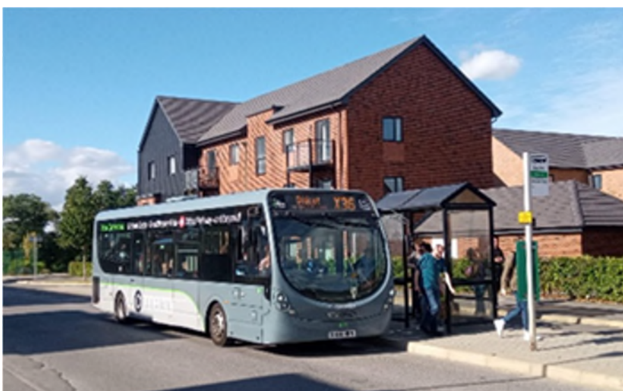
Figure 2 Example of bus infrastructure added to a new residential development.
