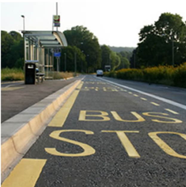
Figure 9 - Example of Kassel Kerb installation
