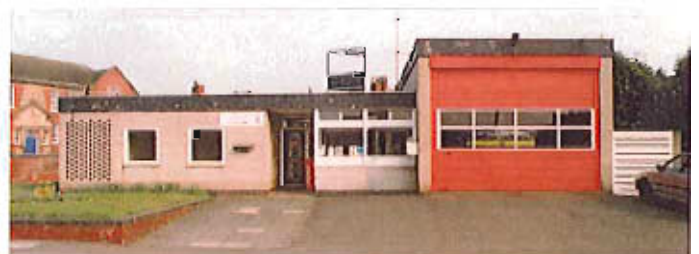
The fire station, built of pale, buff bricks with a flat roof on a distinctly horizontal plane, on the corner of the High Street and Noble Street is equally insensitive to its surroundings.
