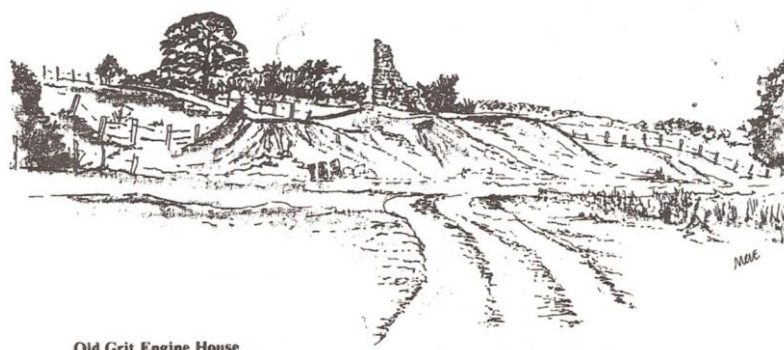
Old Grit Engine House
