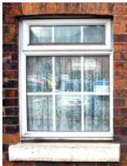
Modern uPVC replacement: This uPVC window is flat, shiny and harsh in appearance. The proportions are ungainly. It appears alien to the historic brickwork around it.
