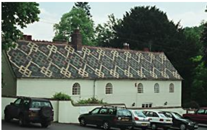
Fig 5.5 Patterned tiling - 20 and 21, Buildwas Road, Coalbrookdale
