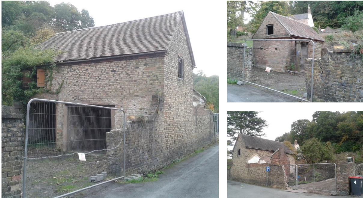
Fig 5.16 Woodside House Barns, Coalbrookdale.
