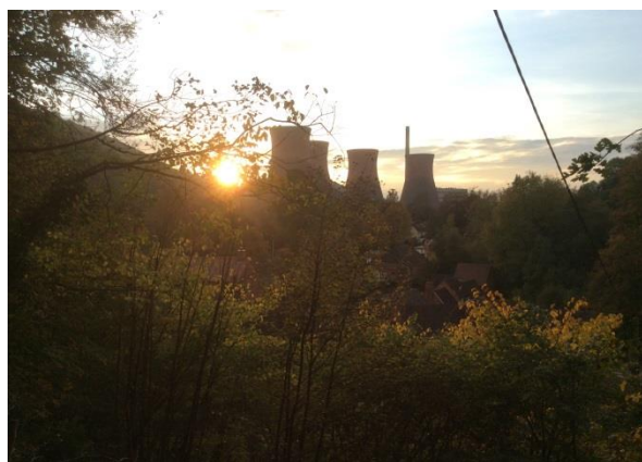
Fig 5.89 View of cooling towers from Lincoln Hill
