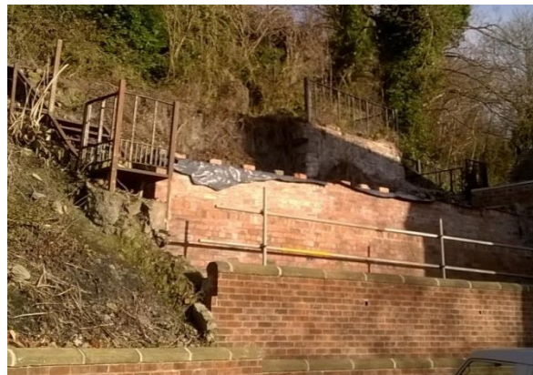
Fig 5.35 Replacement retaining wall after failure of terraced garden. Steep slope impacts on scale of retaining wall.
