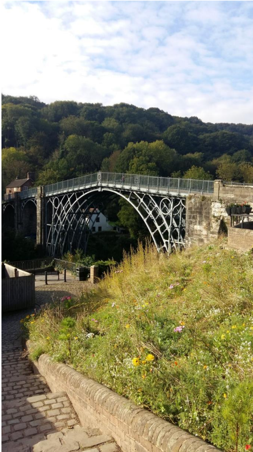
Fig 1.1 View of the Iron Bridge
