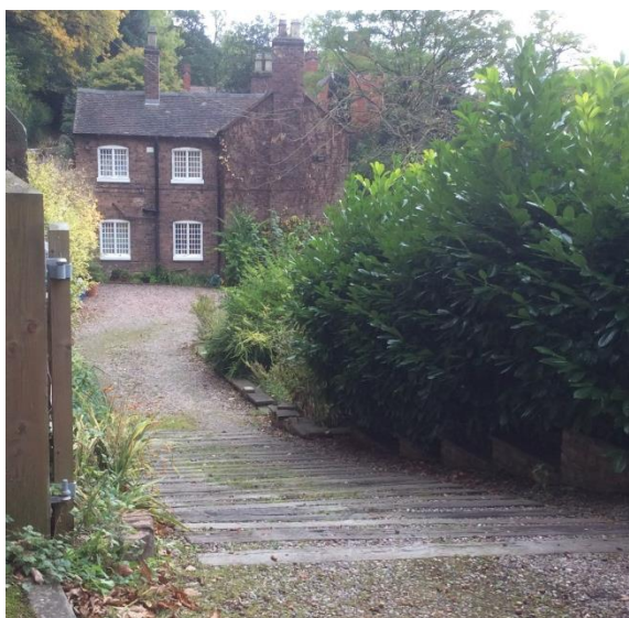
Fig 5.30 clinker/gravel drive with discrete timber sleepers set into slope to stabilise surface, Coalbrookdale
