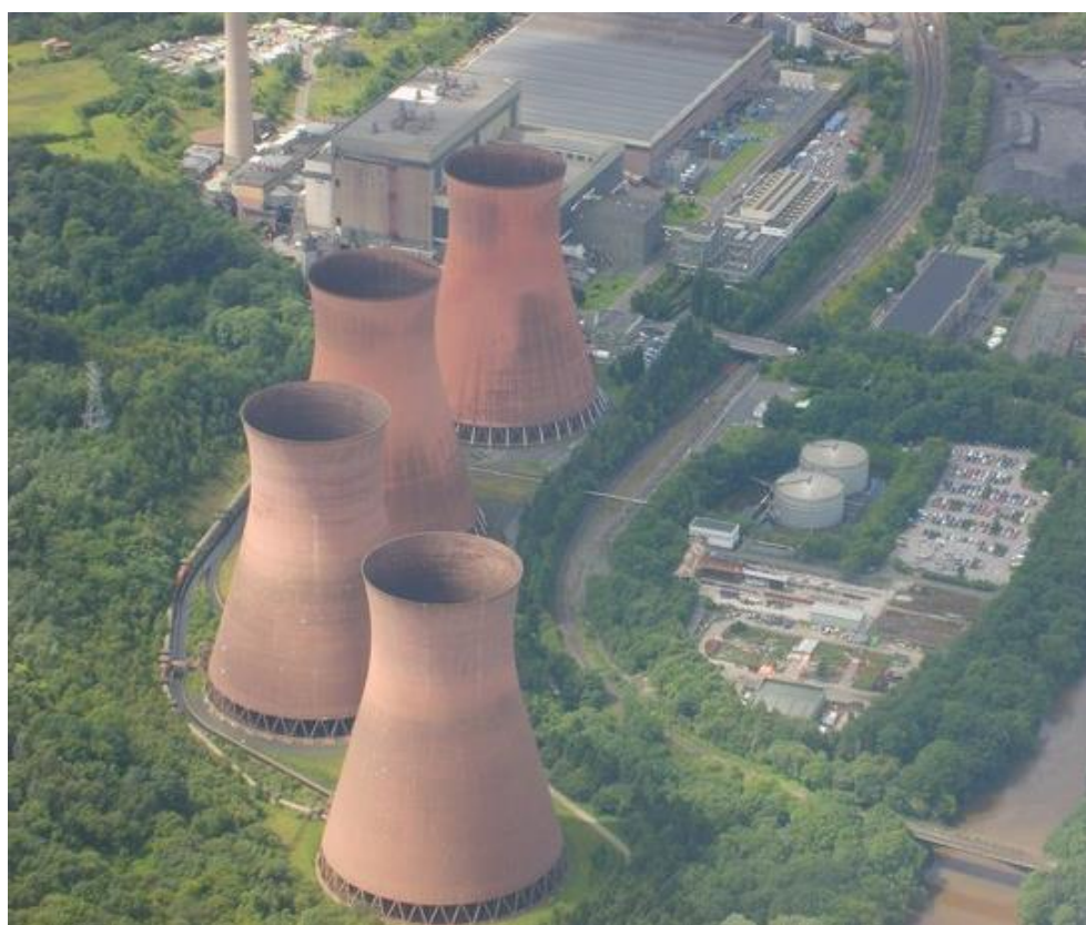
Fig 5.18 Aerial view of Power Station Source: Geograph.org.uk
