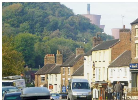
Fig 5.90 View of cooling towers from Ironbridge
