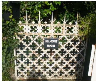
Fig 5.58 Ornate Gothic style gate, Belmont Road, Ironbridge
