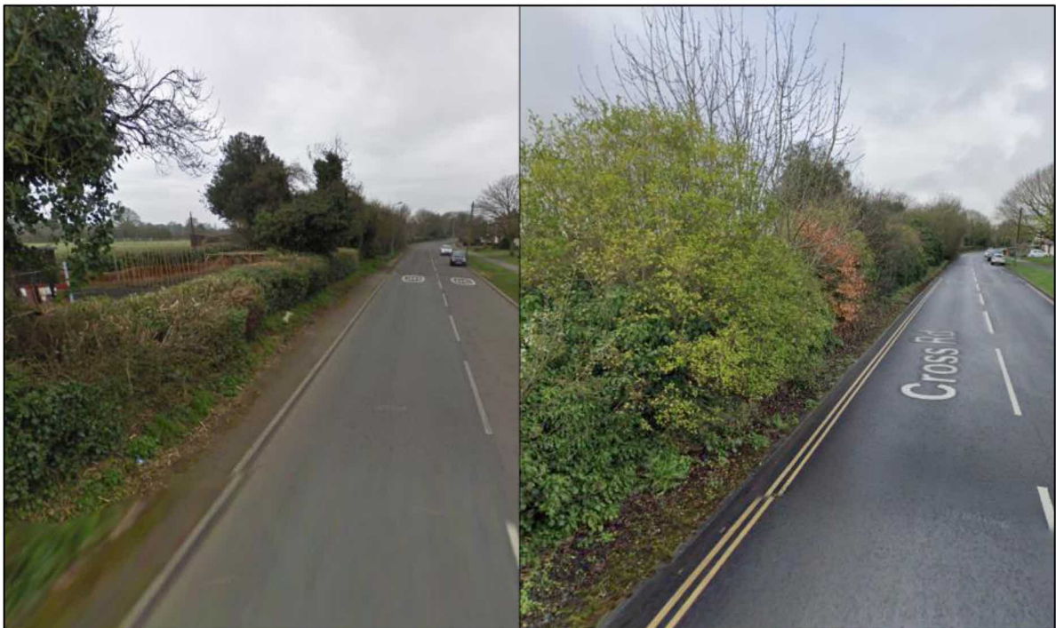
Figure 11. Comparison of Google Street View from 2009 (Left) and 2023 (Right) Showing the Overgrown Footway on the Southern Edge of Cross Road
