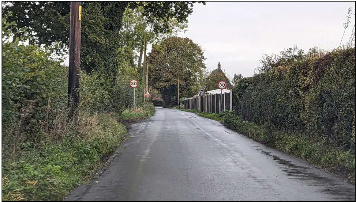
Figure 5. National Speed Limit to 30mph Signage on Patshull Road
