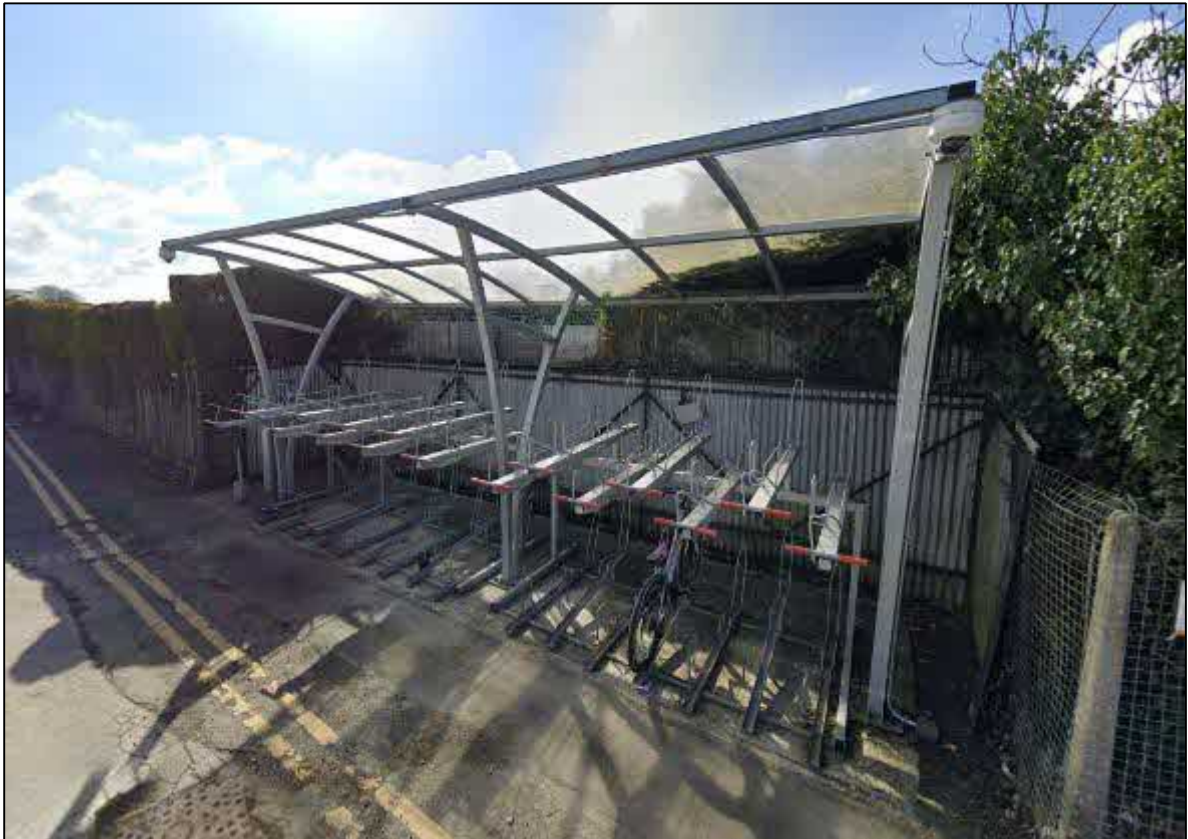
Figure 18. Cycle Parking at Albrighton Railway Station (CCTV Monitored)
