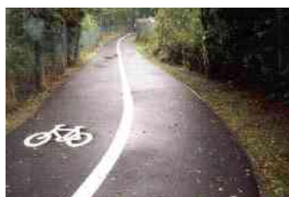
Picture 11.2 Market Drayton footway (after)
