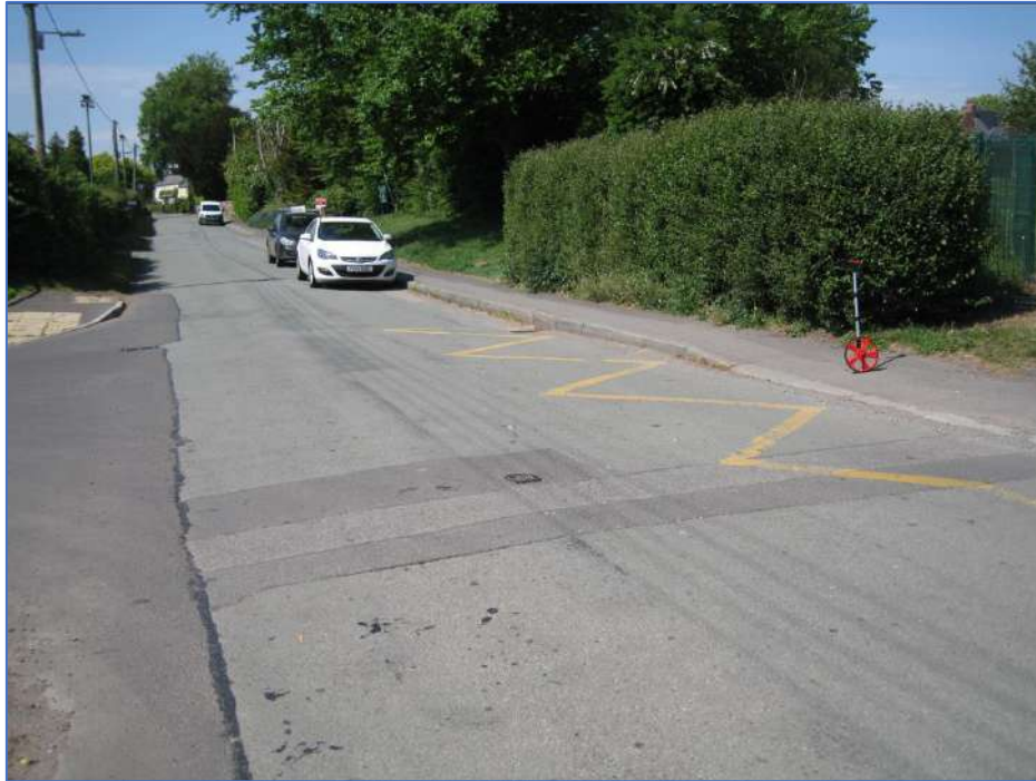
Photo 6 – Tilstock Lane footways west of PROW 0233/28/1
