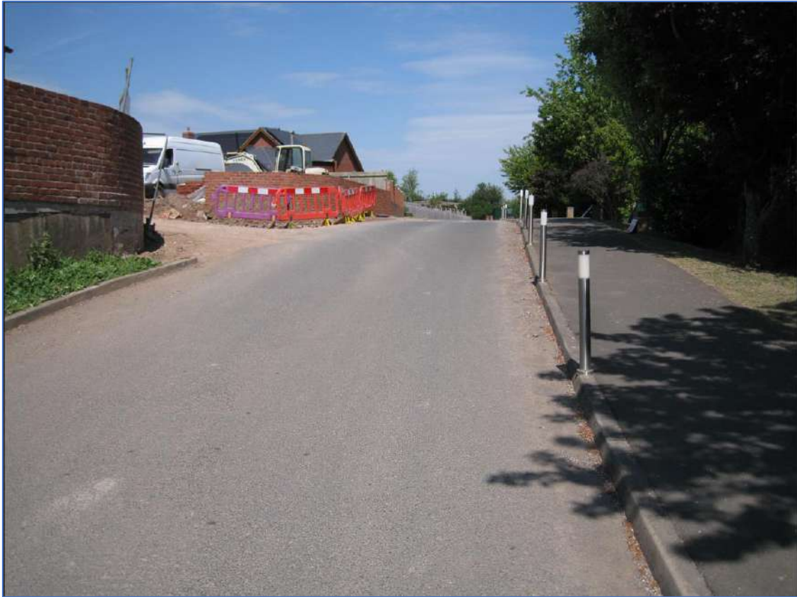
Photo 8 – Footway along eastern side of Crabwell Meadow
