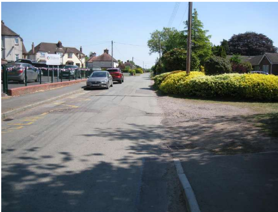
Photo 5 – Tilstock Lane footways east of PROW 0233/28/1
