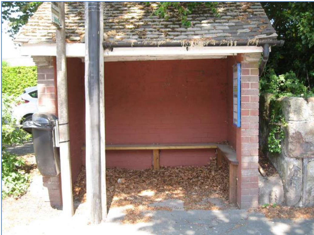
Photo 11 – Tilstock Lane northern side bus stop shelter and seating
