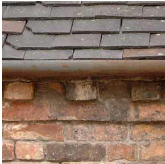
The most common eaves detail is a dentil brick of alternately projecting headers, (left). A moulded brick is used in a few of the better houses, (centre). 43, Darby Road, Coalbrookdale, (right), has a porch made entirely from cast iron.
