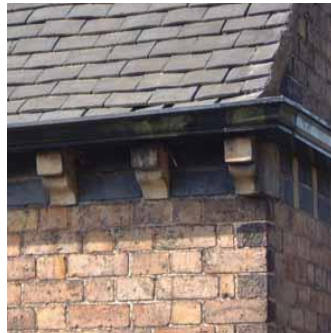
The most common eaves detail is a dentil brick of alternately projecting headers, (left). A moulded brick is used in a few of the better houses, (centre). 43, Darby Road, Coalbrookdale, (right), has a porch made entirely from cast iron.
