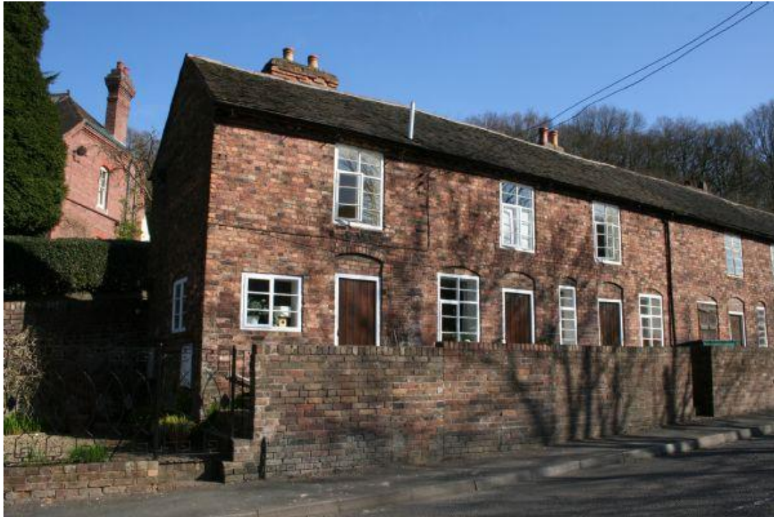
Traditional "ladder" casements in Carpenters Row.
