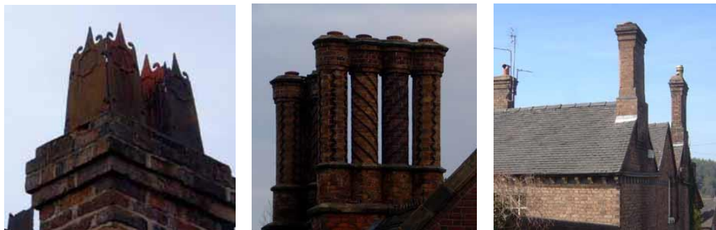
Cast-iron chimney pots are still found, for example at Carpenter's Row, Coalbrookdale, (left). Some of the larger houses have highly ornate chimneys as at Orchard House, Ironbridge, (centre). Chimneys generally are particularly tall, as at Cherry Tree Hill, Coalbrookdale, (right), and form important elements of the profile of built development.
