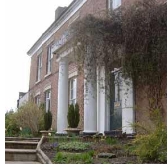
The most common eaves detail is a dentil brick of alternately projecting headers, (left). A moulded brick is used in a few of the better houses, (centre). 43, Darby Road, Coalbrookdale, (right), has a porch made entirely from cast iron.
