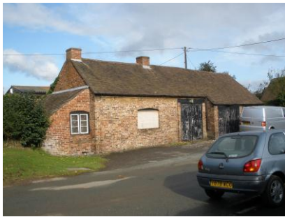
Commercial Unit – Village Road
