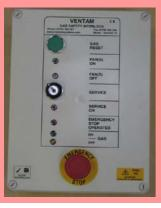
The interlock will shut off the gas supply to these appliances if there is inadequate air movement.
