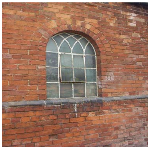
Decorative iron window, Pound Street
