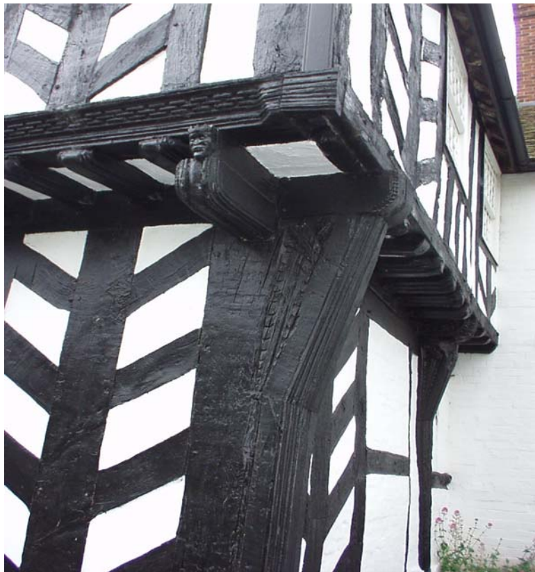
Detail of Jettied first floor at The Vicarage
