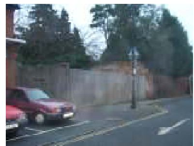
Plate 49: Boundary wall, Town Walls
