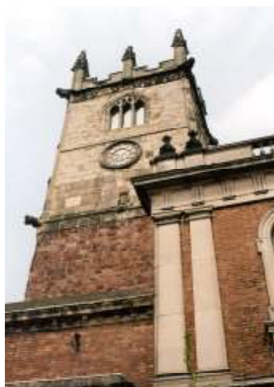
Plate 18: St Julian's Church Tower
