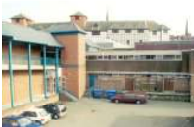
Plate 51: Service Yard, Pride Hill/ Riverside Centre
