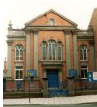
Plate 33: Claremont Baptist Church, Claremont Street
