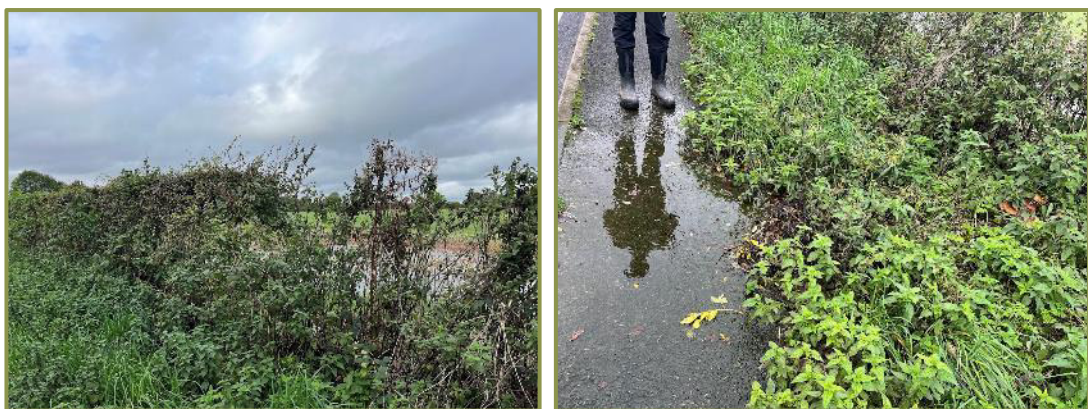
Left: View to the northwest of Surface Water Ponding in the southeast corner of the Site. The ponding is behind the hedgerow. Right: Surface Water Flooding onto the pavement of the A464.
