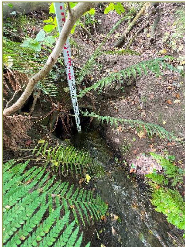
Figure 5.4: Ø600mm Culvert Inlet for Watercourse 3
