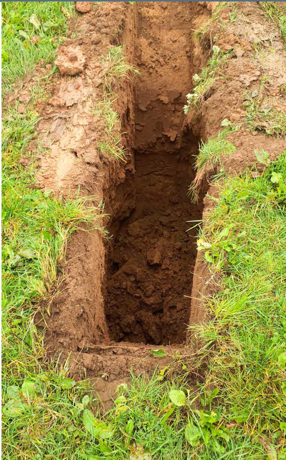
TP06: Showing side wall collapse
