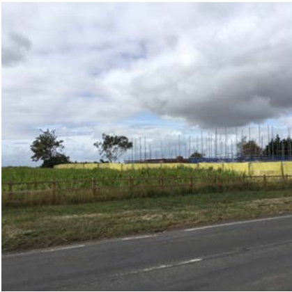
1. FROM A528, VIEW WEST OF BROWNFIELD SITE UNDER CONSTRUCTION
