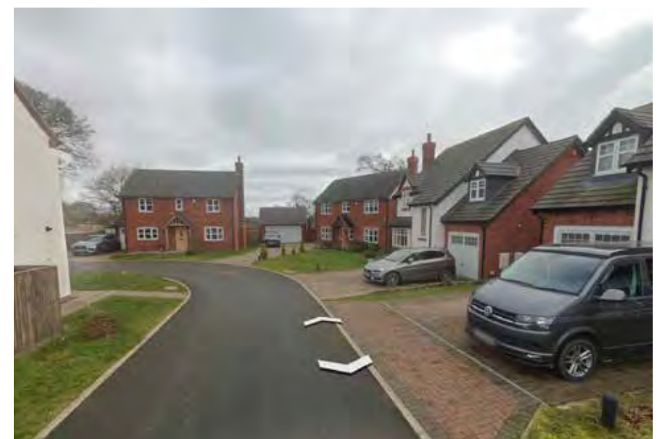
Figure 17: The Pastures, off Tilstock Lane. Source Google Earth
