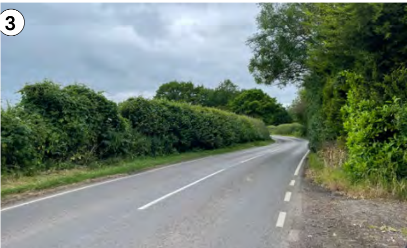
View along the sites western boundary from the B5476
