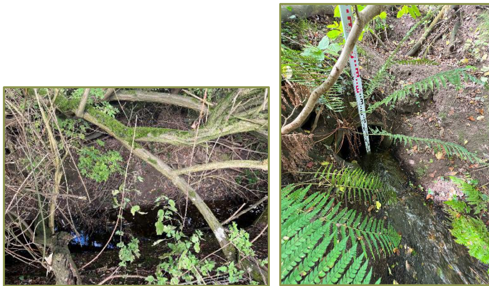
Left: View north of Watercourse 3. Right: Culvert entry and channel depth of Watercourse 3.
