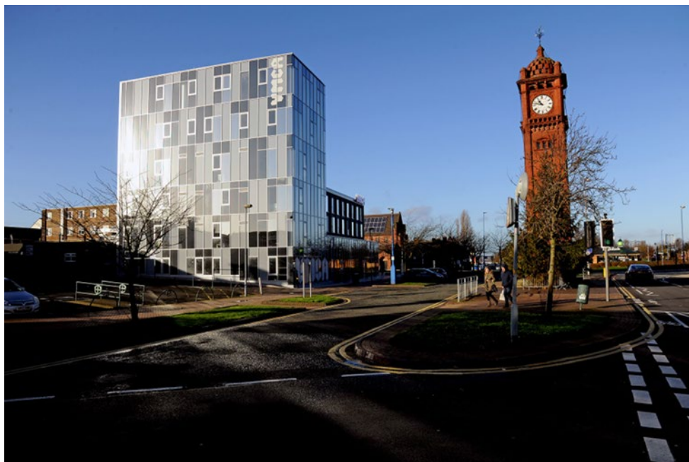
Figure 25. YMCA Western Gateway in West Bromwich
