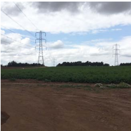
3. OVERHEAD POWER LINE PROMINENT WITHIN THE OPEN LANDSCAPE
