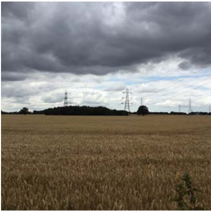
1. OVERHEAD POWERLINES GREATLY DETRACT FROM THE PARCELS VISUAL VALUE
