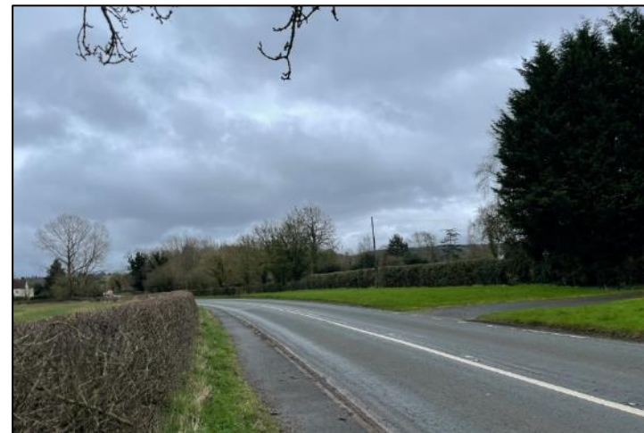
Plate 55: View looking east along Holyhead Road capturing southern boundary of eastern parcel (left) and northern designation boundary (right).
