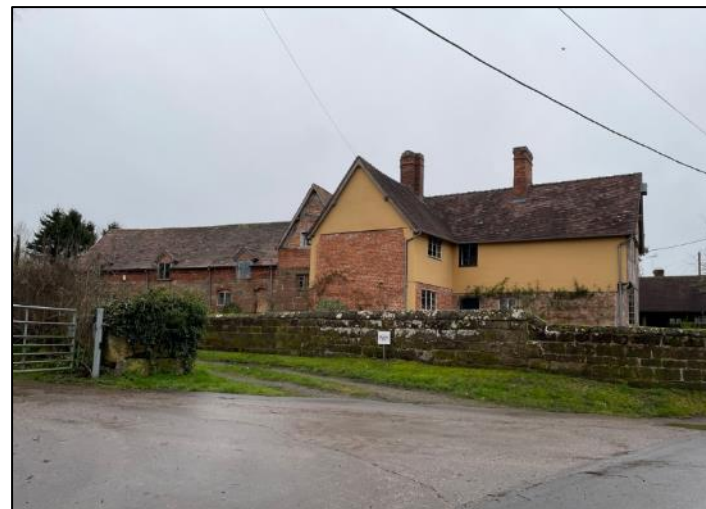
Plate 73: East elevation of Old Farmhouse (right) with attached malthouse (gabled central element) and Grade II Listed Barn (left).
