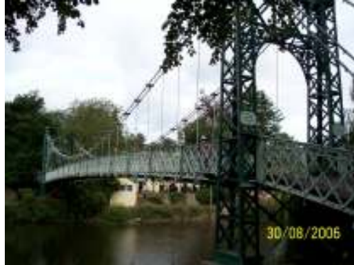
FIGURE 40: Porthill Suspension Bridge
