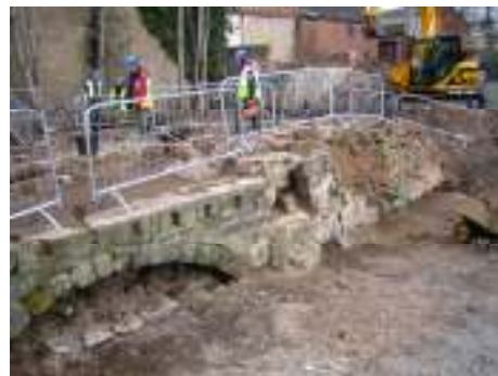
FIGURE 35: The Remains of St George's Bridge
