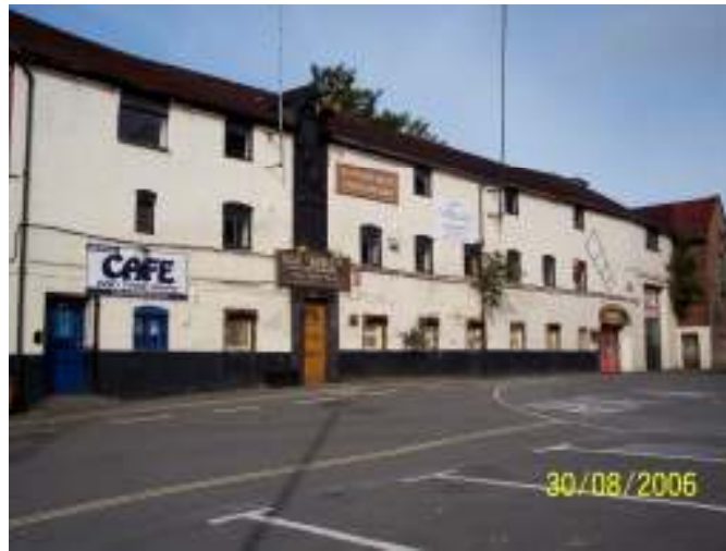
FIGURE 33: The Glen, the largest malting of its time in Shropshire.
