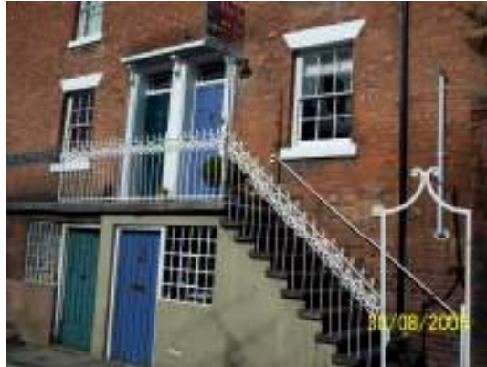
FIGURE 24: New Street, ornate wrought iron railings.
