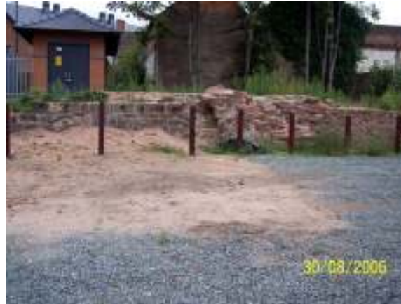
FIGURE 8: Remains of St. George's Bridge, in need of protection.
