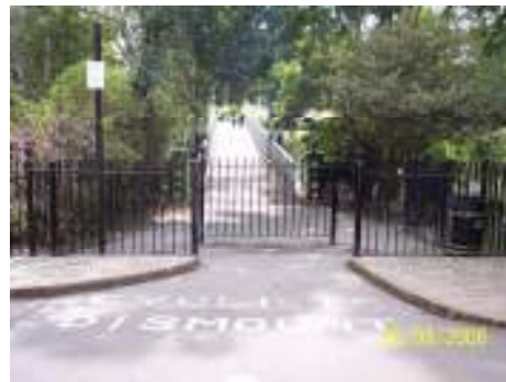
FIGURE 26: Entrance to Porthill Suspension bridge, contrast to existing ornate railings in the area.
